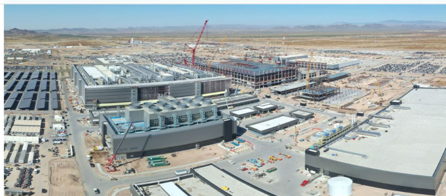
TSMC's Arizona site under construction
